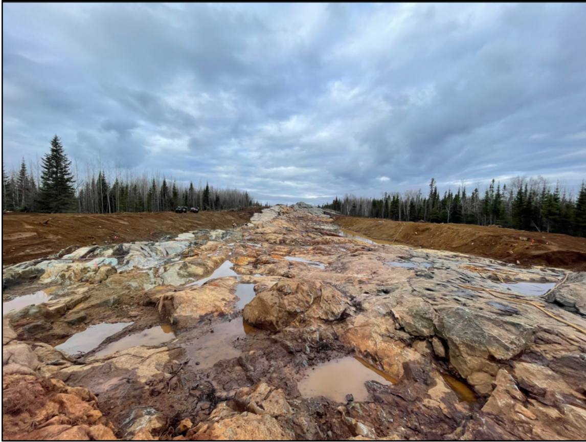
Looking West from Eastern End of Currently Stripped Area
