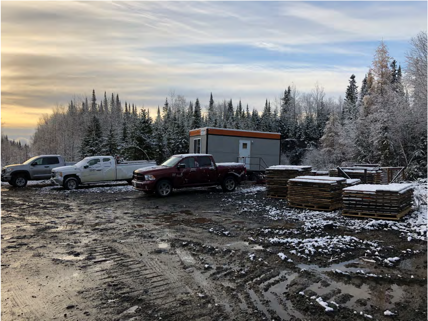
Photo 3: Parbec work site – December 2020
