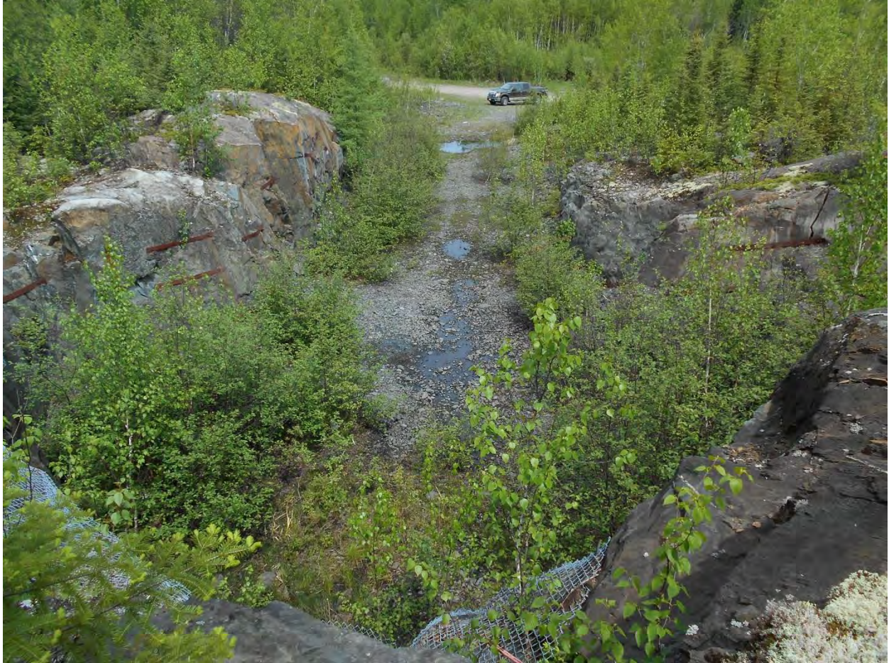
Photo 2 Ramp entrance from above looking northwest
